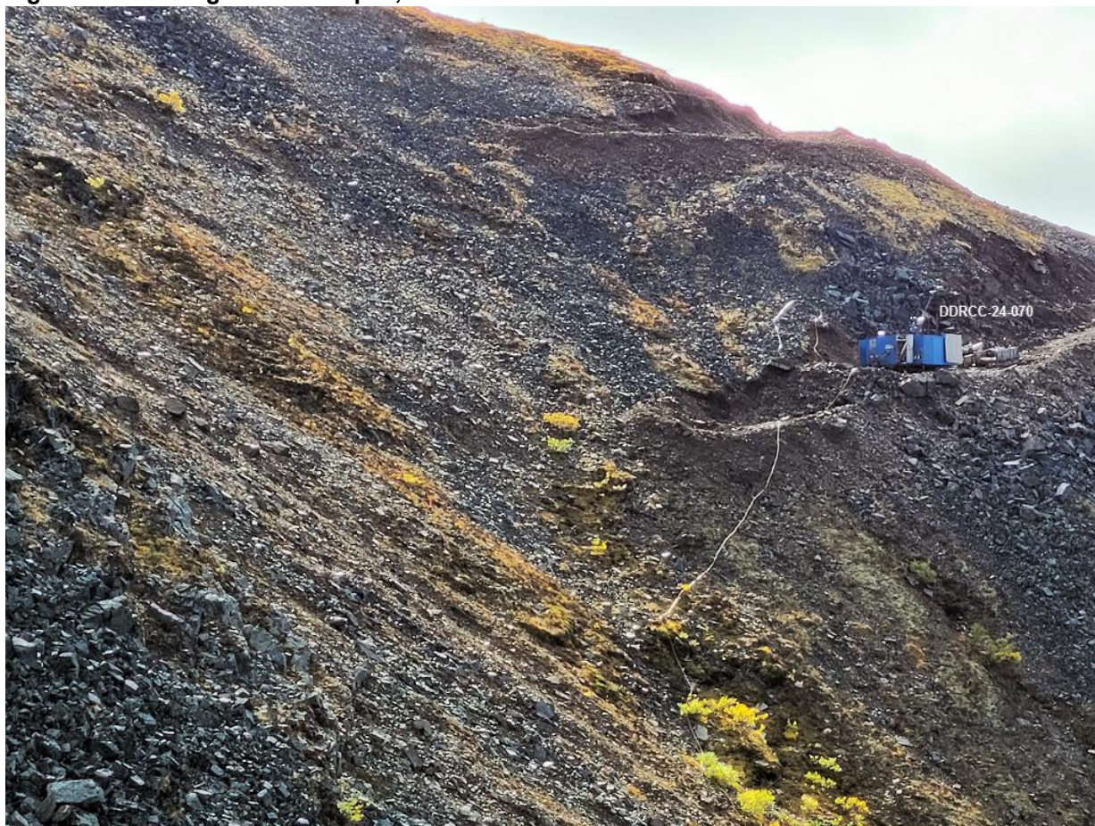
Figure 12-6 Drilling on site - Sep. 5, 2024
